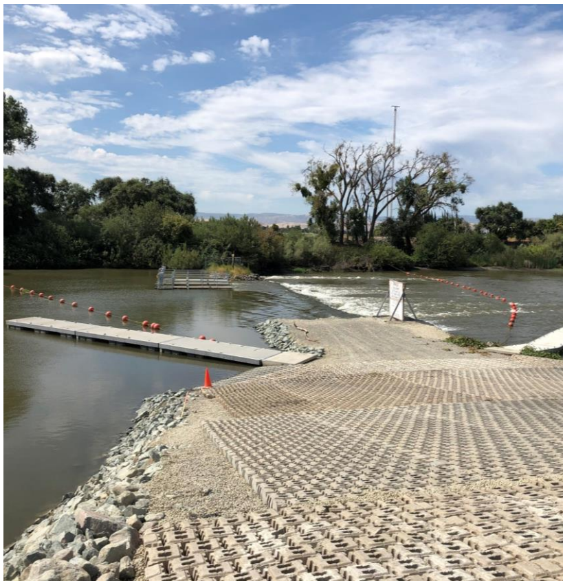
Grant Line Canal Barrier
