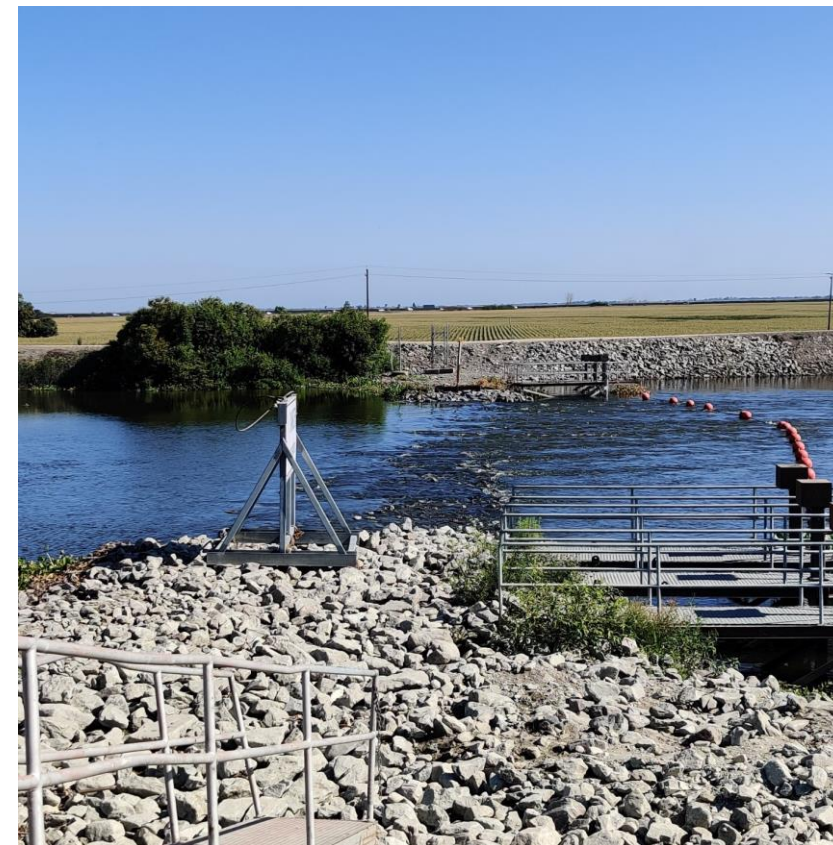
Middle River Barrier
