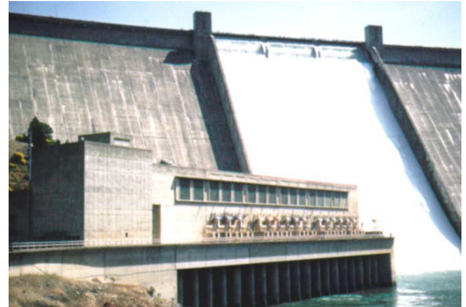
Powerplant at Shasta Dam
