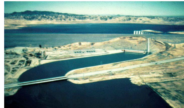
San Luis Power Plant
